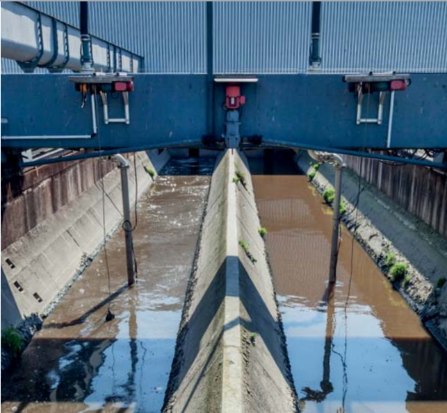
Unbelüfteter Langsandfang
